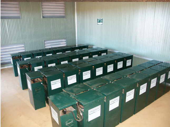
Top: Areal shot of the station and power complex. Middle Left: The solar array and wind turbine. Middle Right: Automatic backup generator. Bottom Left: Deep cycle battery bank in ventilated room. Bottom Right: Instrument/power.
